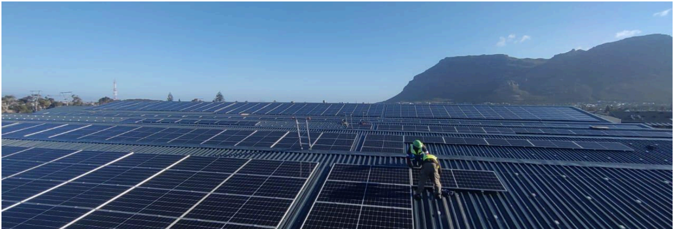
Skills on the roof: local installation teams trained to international standards.
