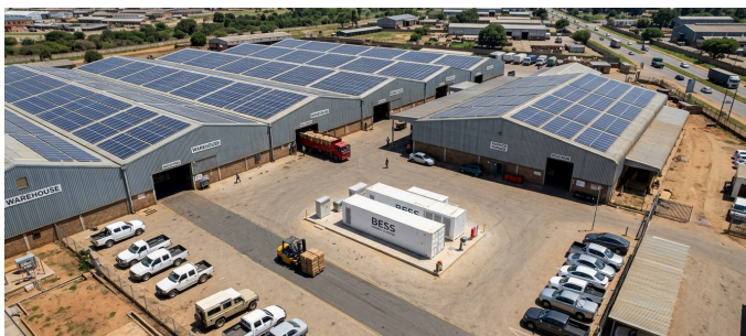
Industrial rooftop solar — Harare, Zimbabwe.
